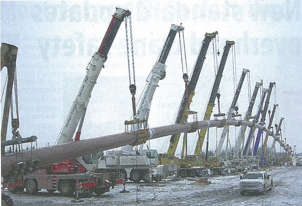
A line of Liebherr and Grove 100- to 165-ton all-terrain cranes supplied by NCSG Crane & Heavy Haul attend to a pipeline pull in Alberta. The 42-inch pipe was lifted so it would be at the right angle to be pulled underneath a river in Alberta.
