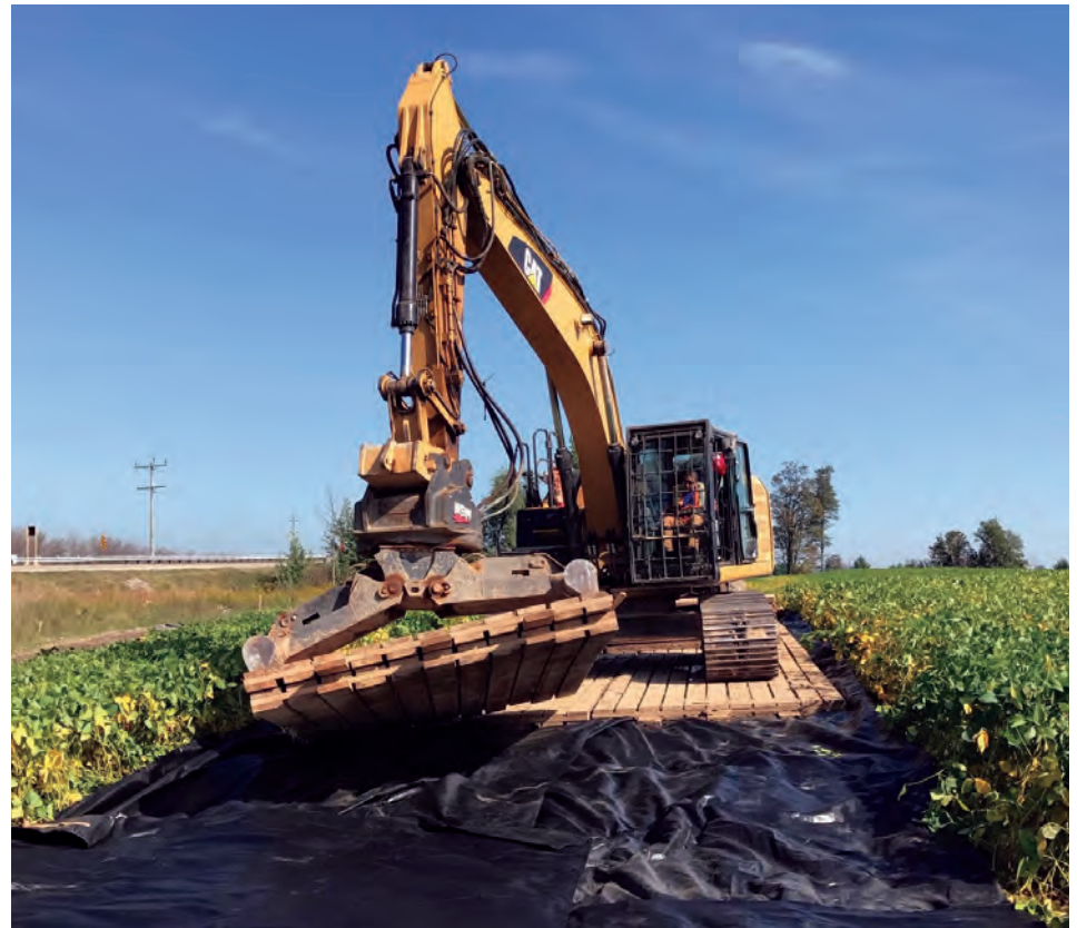
Member Tyler Longboat installing mats with Northern Mat and Bridge.
